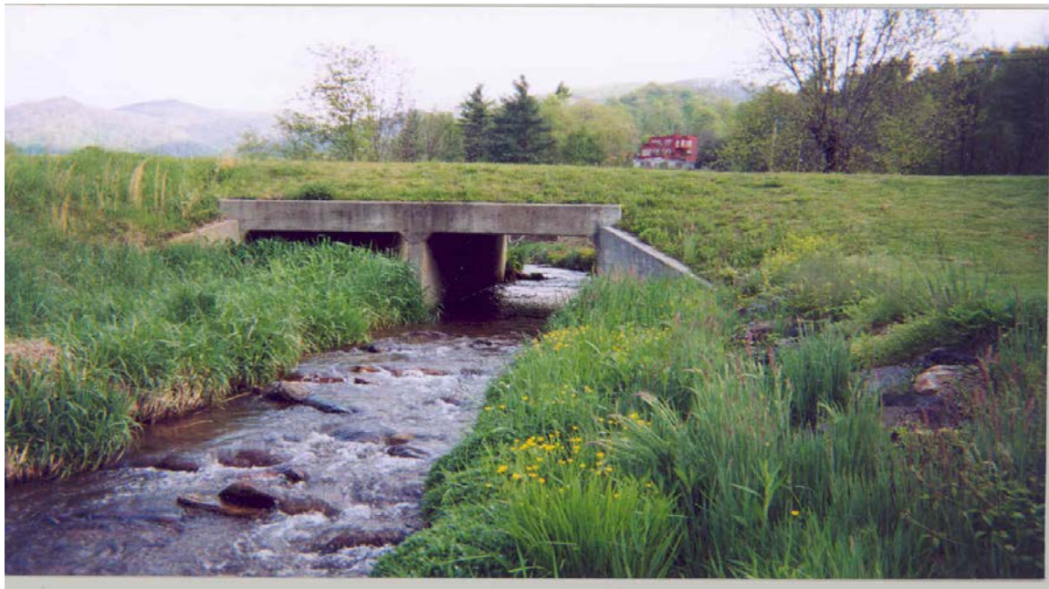
Figure 4-Culvert with floodplain bench
